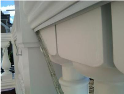
Using IlluminFx track (p/n T13-3, seen on the underside of the porch railing) is a simple way to mount LED rope light to the desired location. Epoxy and/or screws can be used to secure the track in place, and then the rope light can be snapped into the track. (Note: T13-3 track is clear. The track in this figure has been painted.)
