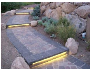
Lighting path steps.
