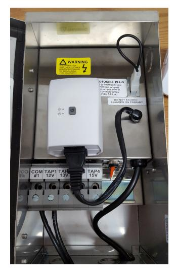
This shows the correct wiring using 12AWG going out of the transformer to the lighting fixtures. As well as the
